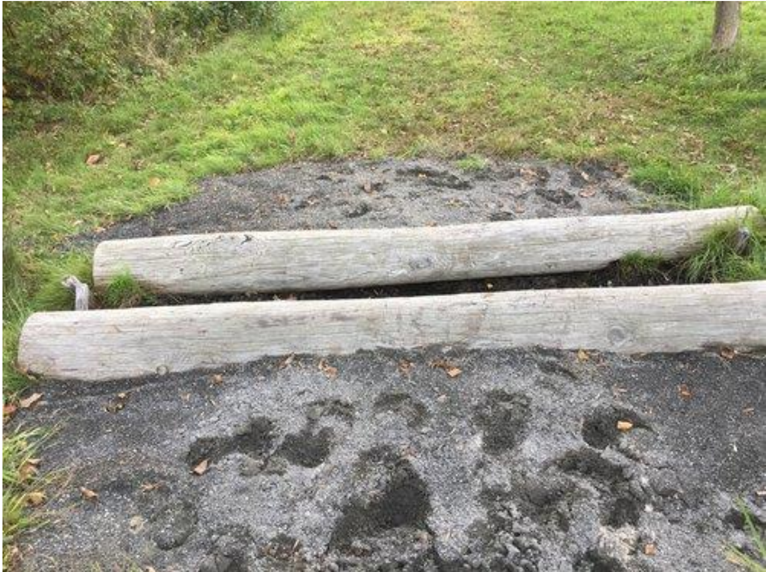
08 Echos Almost A Ditch
